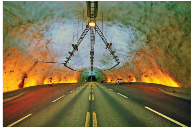
Mood lighting and laybys inside Norway's Lærdal Tunnel. Photo Kristinn Einarsson
